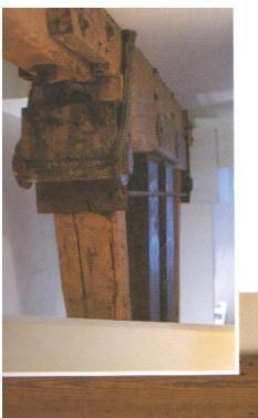
LEFT The massive slabs of timber that supported the winch are studded with bolts, cracked and dented by years of use. The slim lines of the glazing bars on the windows upstairs look all the more dainty in their rugged company.
